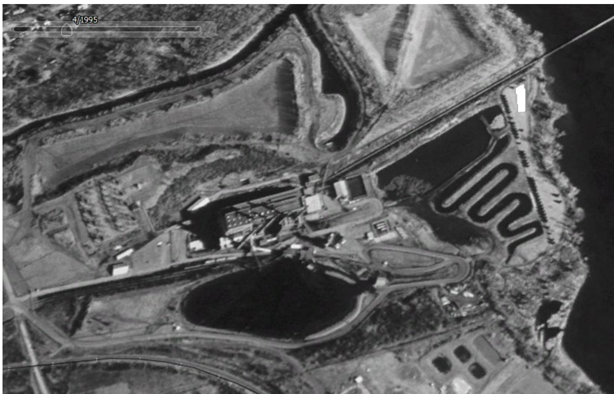
Figure 3 Aerial photograph of the Greenidge site from April, 1995. Imagery obtained from Google Earth on 2/25/22.
