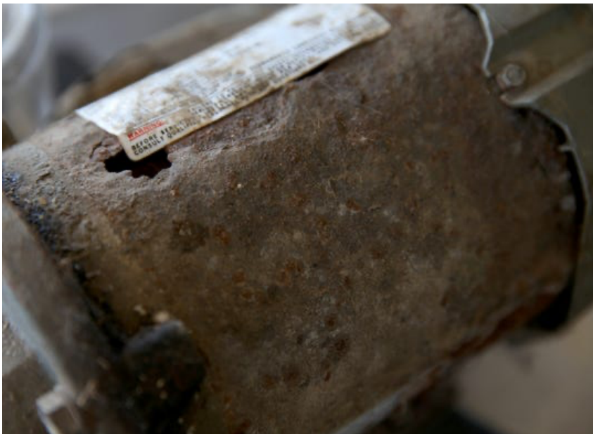
A pump on the Frederick Farm in Phelps that they believe was corroded by salts in the water (2016 photo) (Photo: File photo/Max Schulte)
