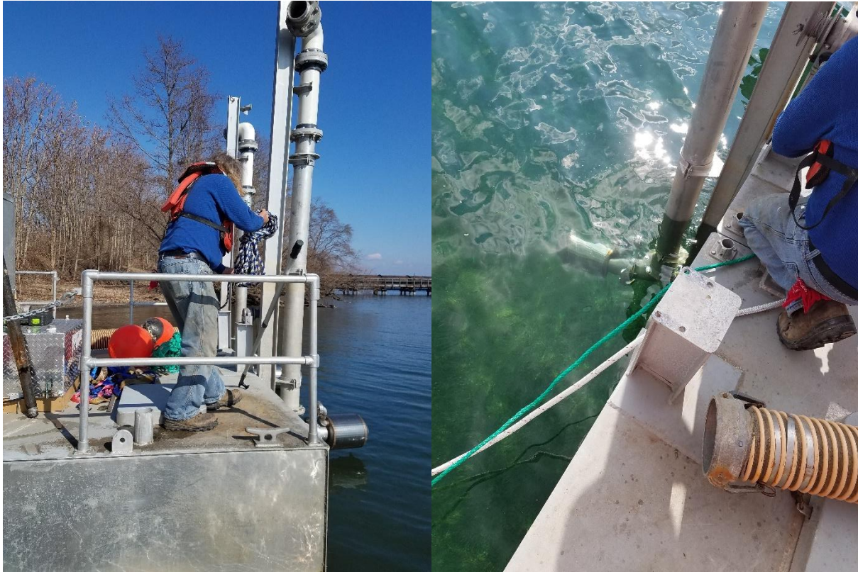
Figure 3-5 Intake end of barge showing intake screens raised (left), and with screens deployed, showing clarity of water in Seneca Lake at time of deployment in March, 2019.
