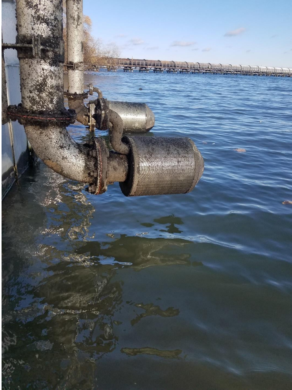
Figure 4-6 State of intake screens when raised for demobilization at end of the 2019 CWWS Pilot Study.
