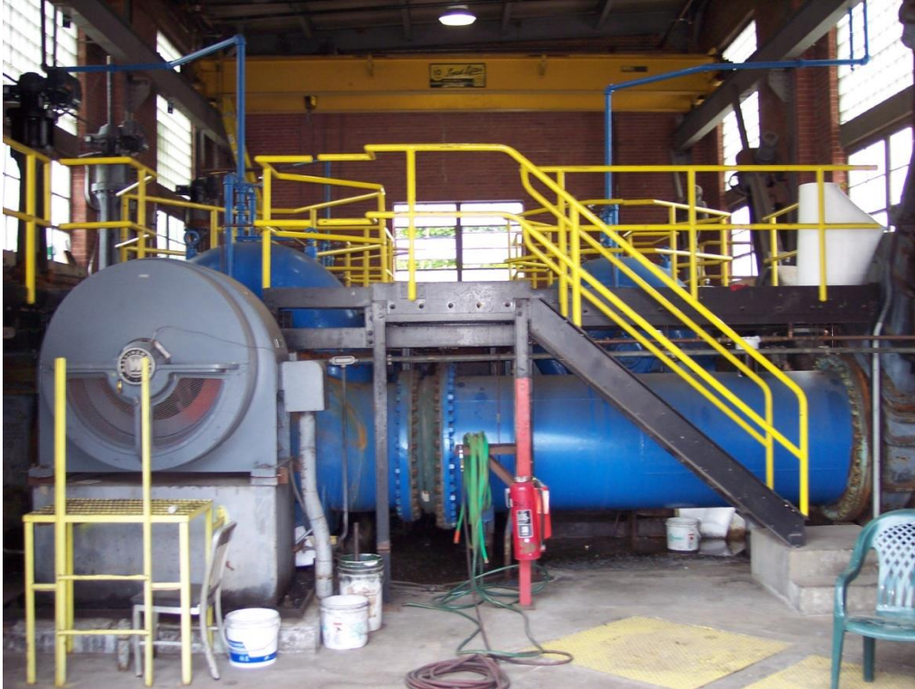
Figure 2-3 Greenidge Unit 4 circulating water pump A.
