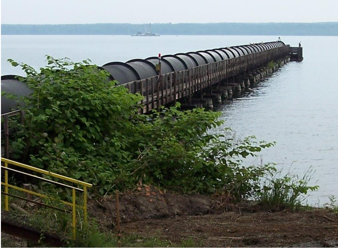
Figure 2-2 Greenidge Generation Unit 4 intake pipe
