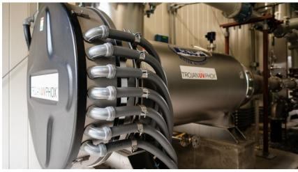
The Suffolk County Water Authority's Advanced Oxidation Process treatment system, designed to remove the contaminant 1,4-dioxane from groundwater, at the SCWA Commercial Boulevard pump station in Central Islip in December 2018. Photo Credit: Barry Sloan
