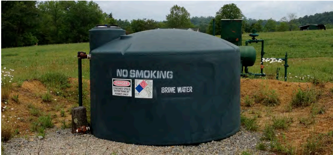
Brine storage tank. Photo by Nadia Steinzor.
