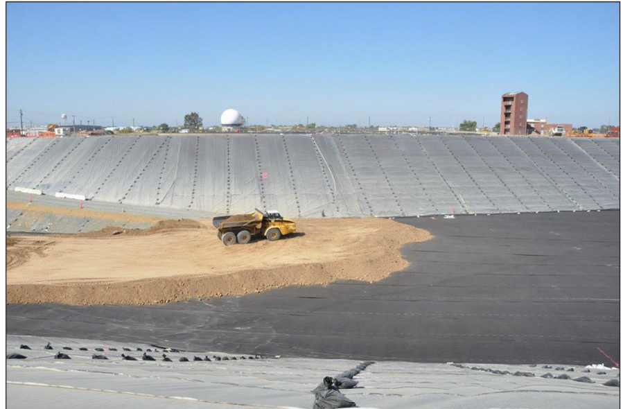
Figure 4: Consolidation Landfill at Former McClellan Air Force Base, California
