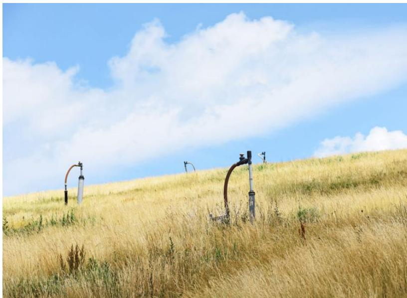
Pipes collect landfill gas to be converted into energy at Seneca Meadows.
