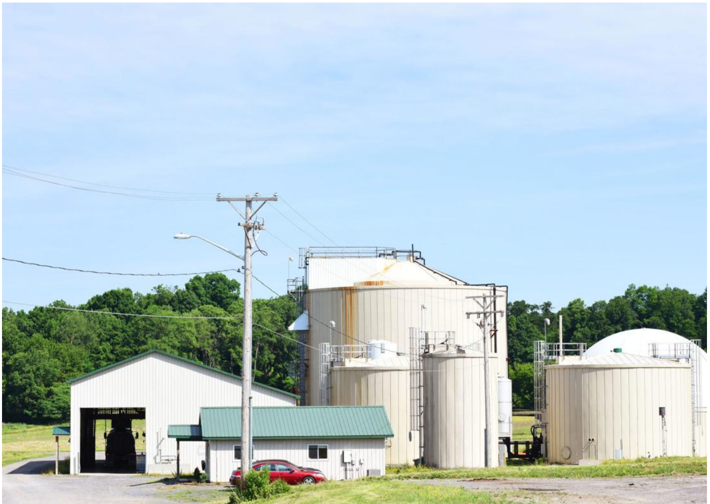
The Cayuga County digester in Sennett.
