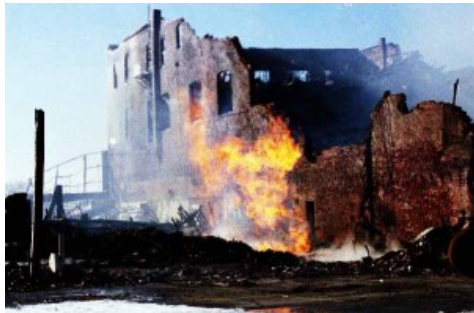
This fire that followed natural gas explosions in downtown Hutchinson, Kan., in 2001 was traced to gas leaks from a salt cavern storage facility seven miles away.
